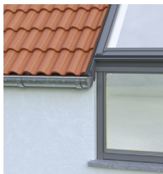
Flush dakrand detail
